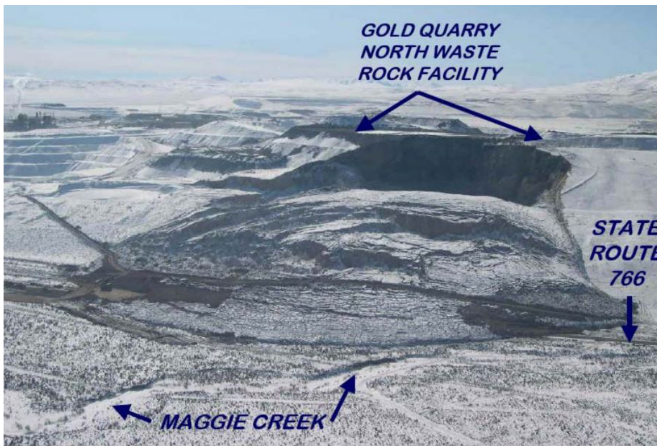
Runout zone of waste rock failure at the Gold Quarry Mine (see footnote 16).
